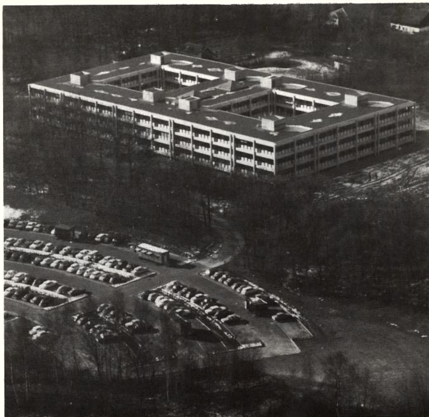
Headquarters of Chief of Defence Denmark in Vedbæk North of Copenhagen.
